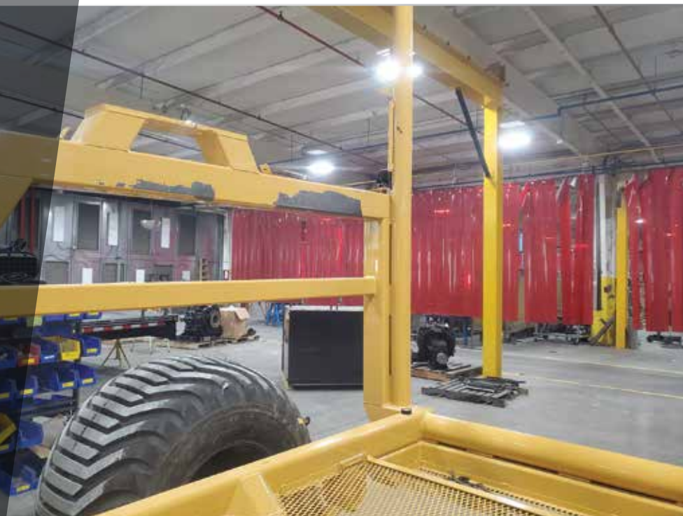
Sections of the topcoat and primer were peeling off, exposing the steel substrate.
